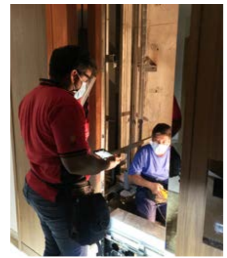
Inspection of lift maintenance works.
